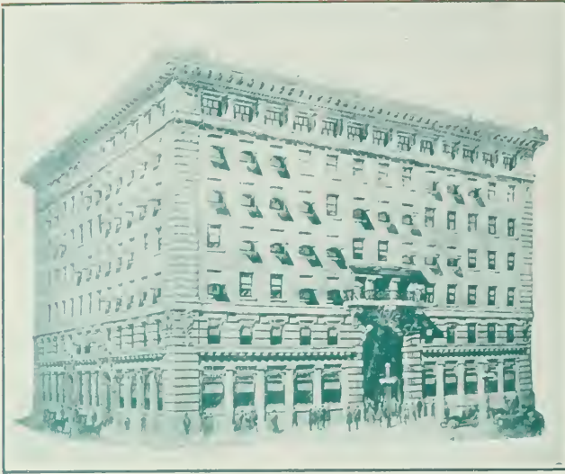
GRAIN EXCHANGE, WINNIPEG Finished with "Empire" Cement Wall Plaster
